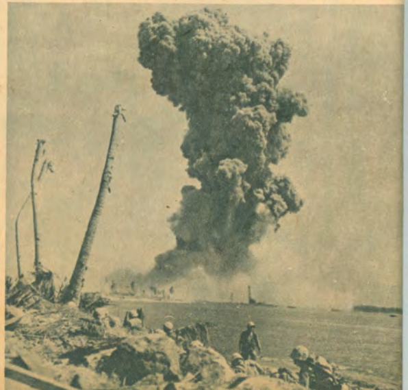
16 —Jap installations on Namur go sky-high as Marine demolition squads go into action. On close-by Roi Island beach (in the foreground) more Marines return enemy sniper fire.
