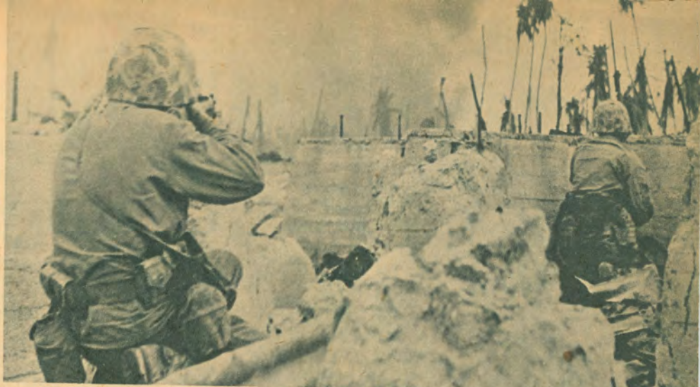
8—Two Leatherneck sharpshooters take cover behind the blasted foundations of a Jap building to pick off snipers. Smoke (background) is still climbing skyward from a fuel dump set off during the bombardment.
